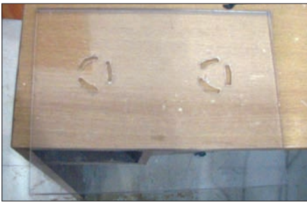
Cut out circular pieces to allow air flow
